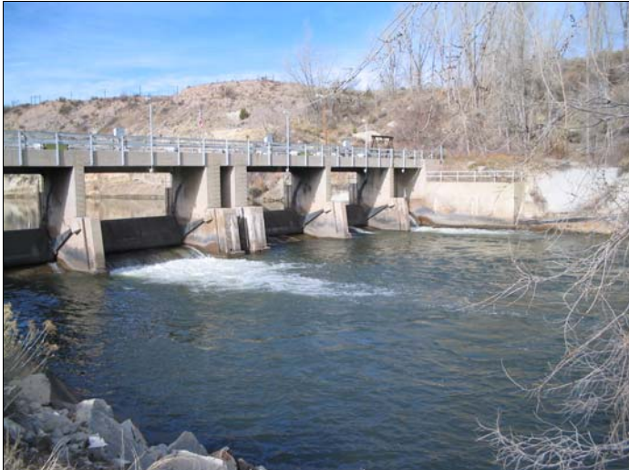
Headworks of the Minnequa Canal on the Arkansas River
