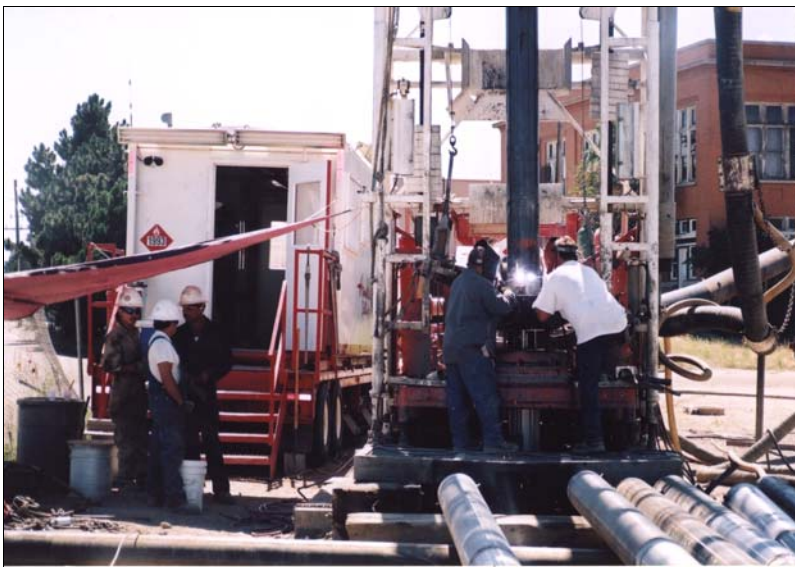
Construction observation during casing welding operation at a typical well
