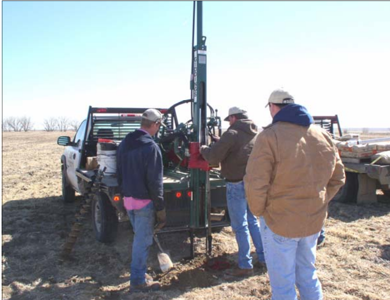
Monitor well installation
