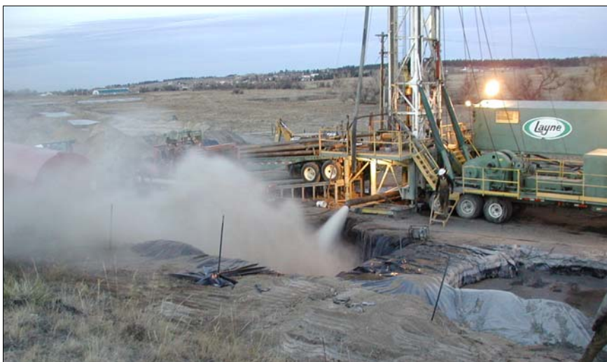
Airlifting water from McLain Well A-1
